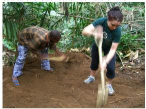
storage tank site is dug out with a fairly level floor. Tomorrow we'll put sand in to level it.
