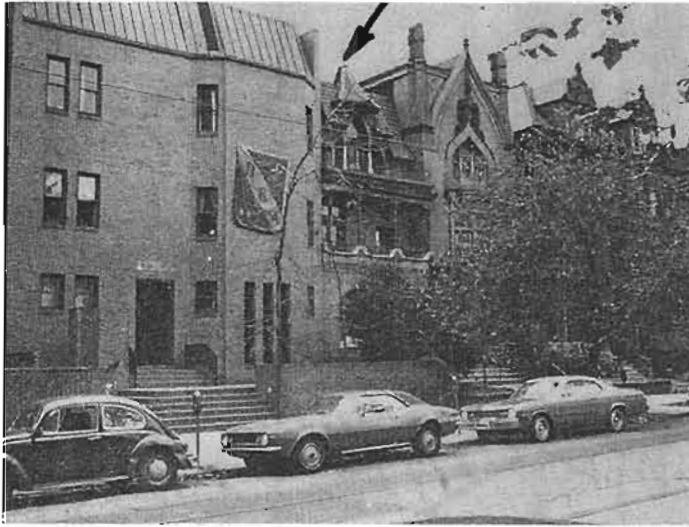
FIG. 1 Solar Retrofit House 3920 Spruce Street View Looking South
